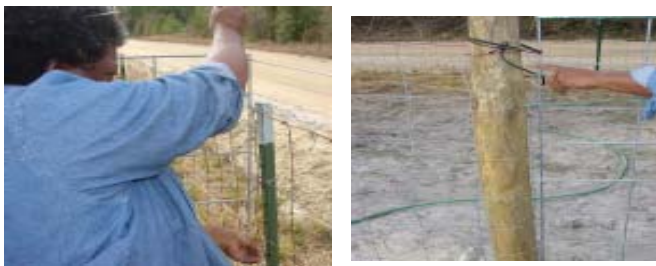
Fig. 11 Use nylon rope to secure the panel to the post.
